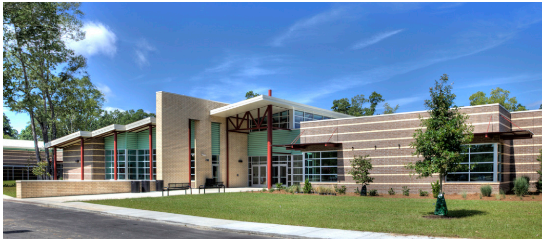
View of Front Entry/Auto Drop-Off
