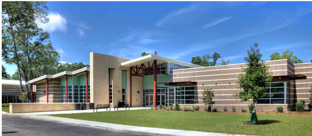
View of Front Entry/Auto Drop-Off
